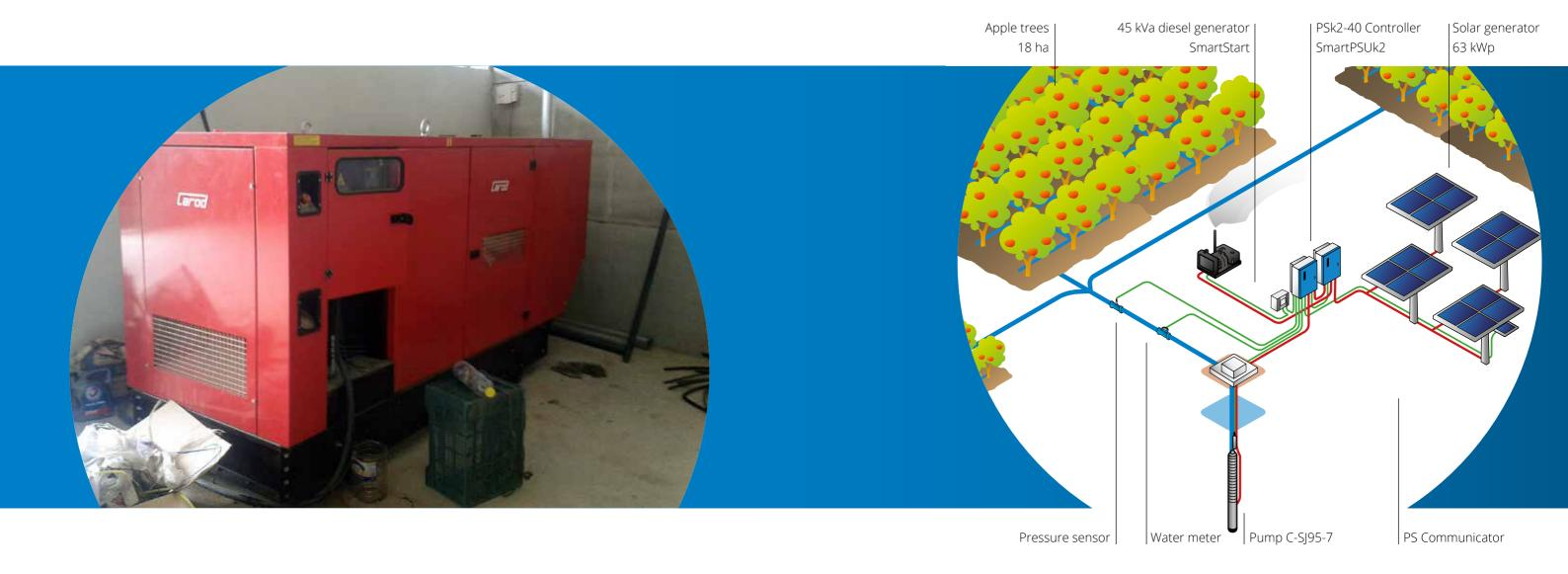
A substantial part of the operating costs are in running and maintaining a large AC water pump powered by a 200 kVA diesel generator to irrigate the apple trees. As the cost for fossil fuels will rise and the fruit market is price
